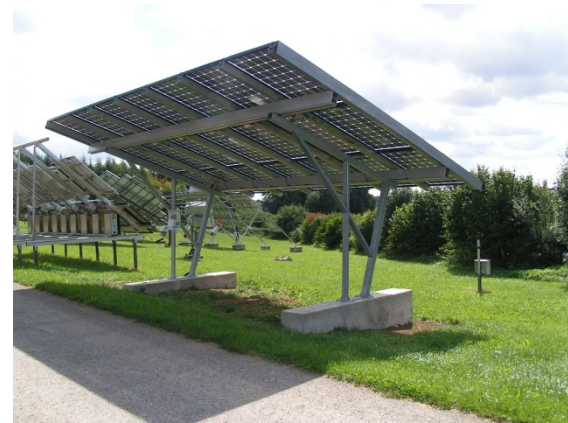
Figure 2: The PV Generator of the Sol-Ion installation at ZSW Widerstall consists of 21 modules (Galaxy Energy GS245m) with nominal 5.145 Wp mounted on a double carport.
